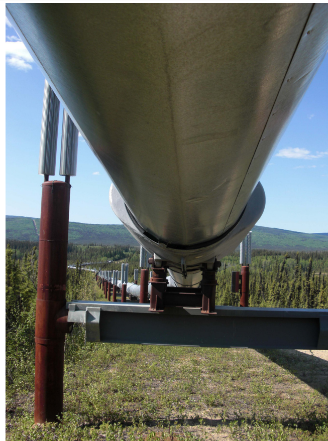
Trans-Alaska Pipeline at Fox, Alaska
