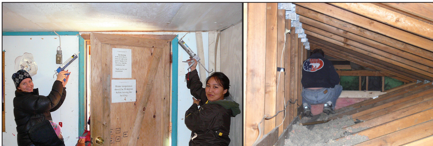
Left: Caulking the Nightmute Community Hall. Right: Insulation being installed into a roof space of a residence in Fairbanks.
